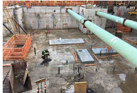
Cellar level at 600 W. 125th Street
