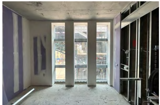
The third floor at 600 W. 125th Street
