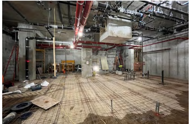
The cellar of 600 W. 125th Street
