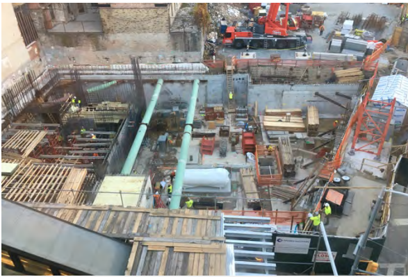
600 W. 125th Street, looking west
