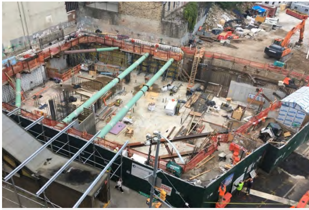
600 W. 125th Street, looking west
