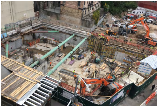
600 W. 125th Street, looking west
