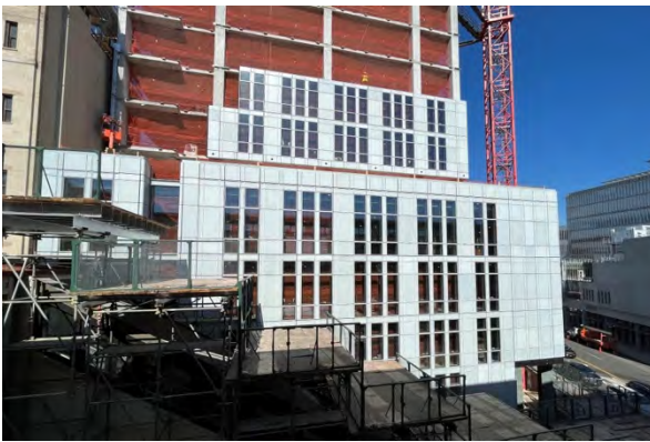
600 W. 125th Street, looking west
