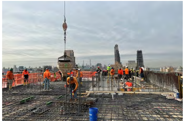
The 22nd floor at 600 W. 125th Street
