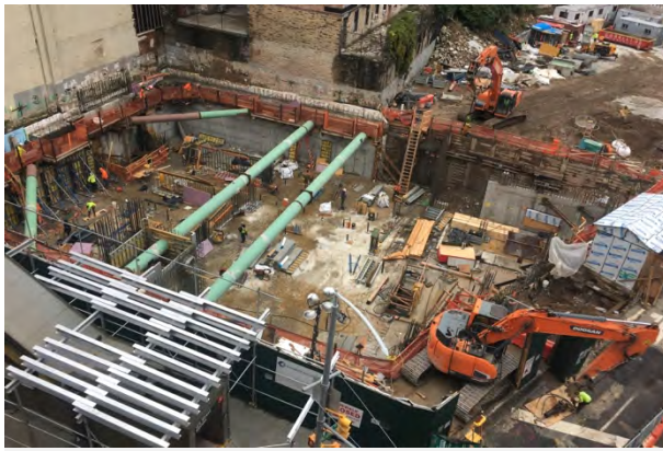
600 W. 125th Street, looking west
