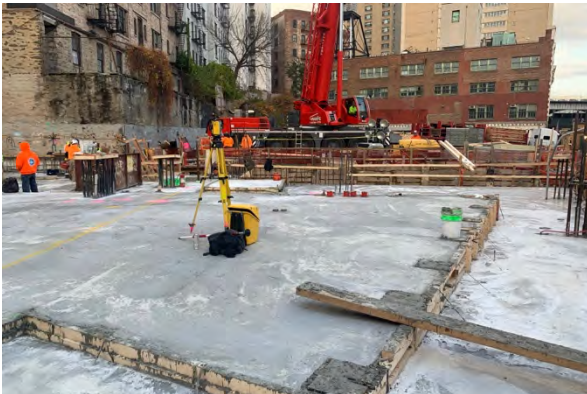
600 W. 125th Street, looking west
