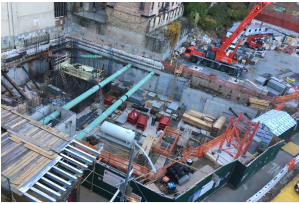
600 W. 125th Street, looking west
