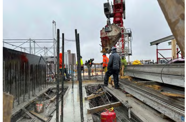
Concrete pour of the 20th floor at 600 W. 125th Street
