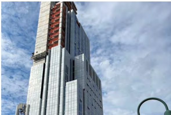
600 W. 125th Street, looking northwest
