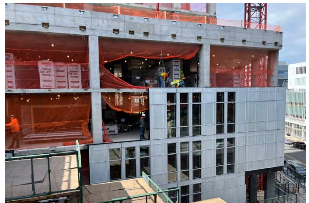
600 W. 125th Street, looking west
