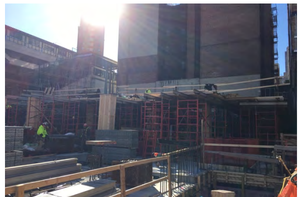
Formwork supporting the second floor at 600 W. 125th Street
