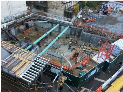
600 W. 125th Street, looking west
