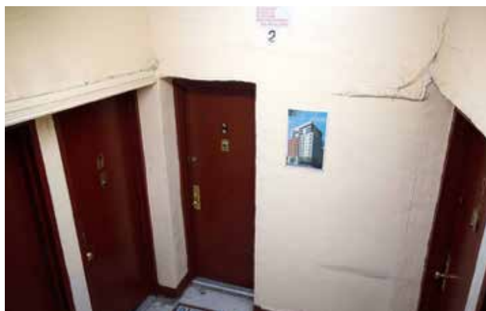
A photo of the new building hangs in the hallway of the 132nd Street structure that will be razed.
