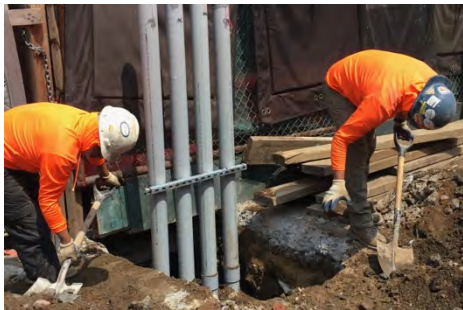
Temporary power conduits at 600 W. 125th Street
