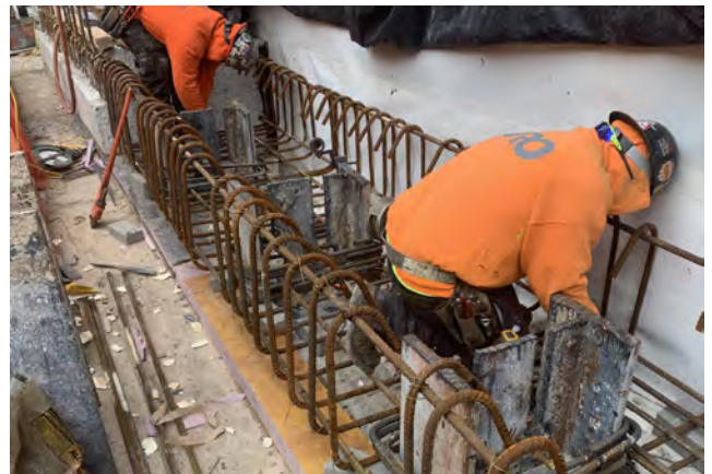
Capbeam installation at 600 W. 125th Street
