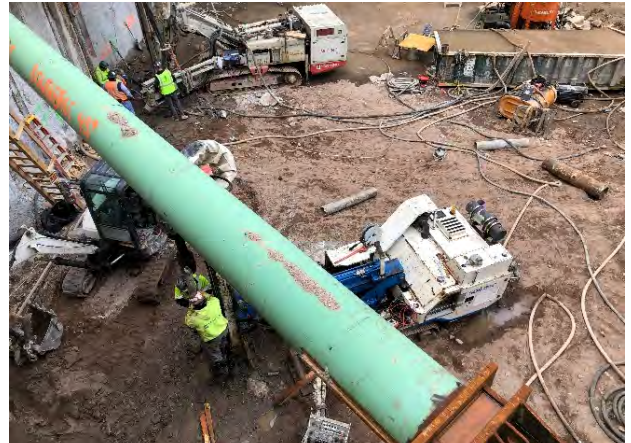
Tangent pile drilling
