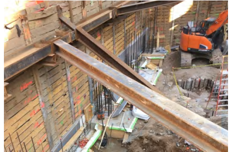
Footing Rebar Installation at 600 W. 125th Street
