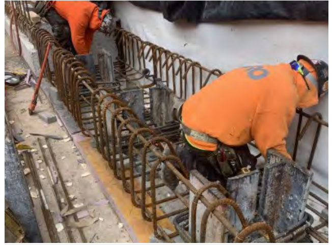
Capbeam installation at 600 W. 125th Street
