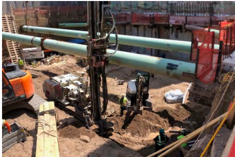
Installation of dewatering system at 600 W. 125th Street
