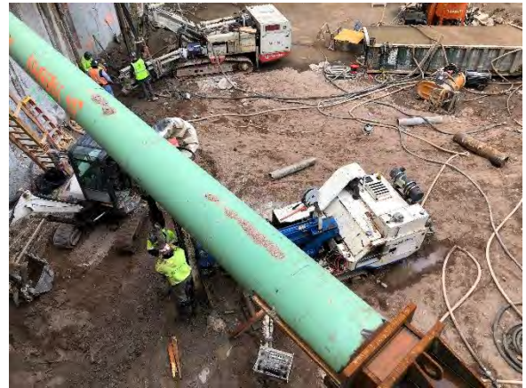
Tangent pile drilling
