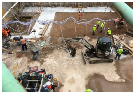
Elevator pit and dewatering system at 600 W. 125th Street
