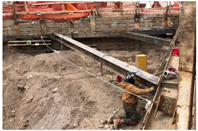
Corner bracing performed at 600 W. 125th Street
