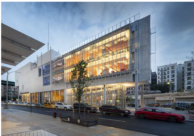
The exterior of The Forum was designed to accommodate the functions of the building — a prefabricated concrete skin provides opacity for its auditorium, and a glazed façade allows daylight to illuminate the office spaces. (Photo: ©Nic Lehoux)
