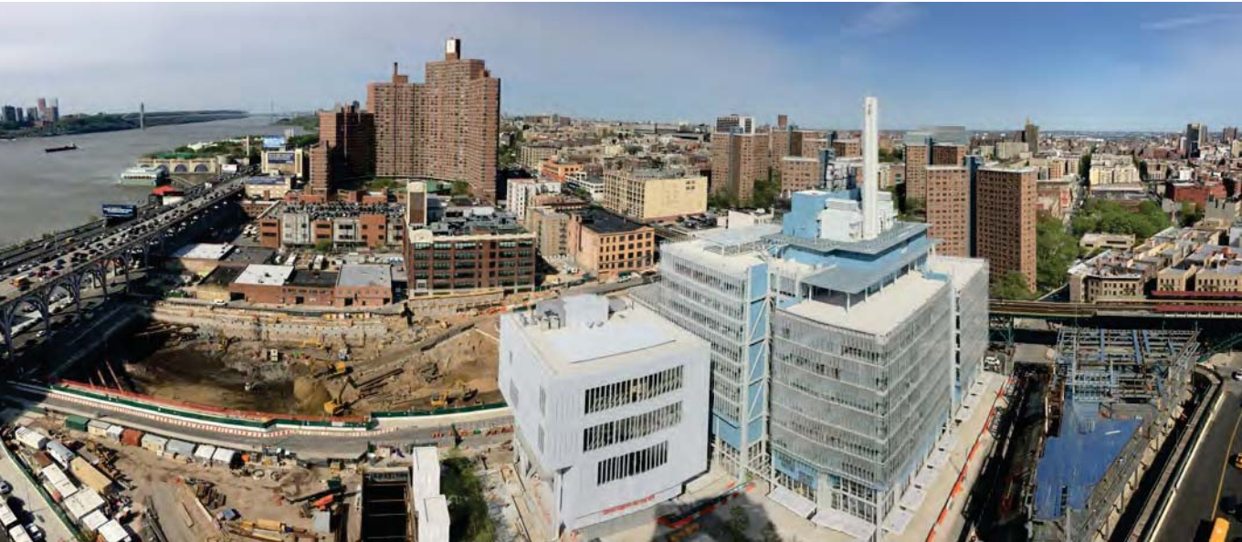
Aerial view looking northeast
