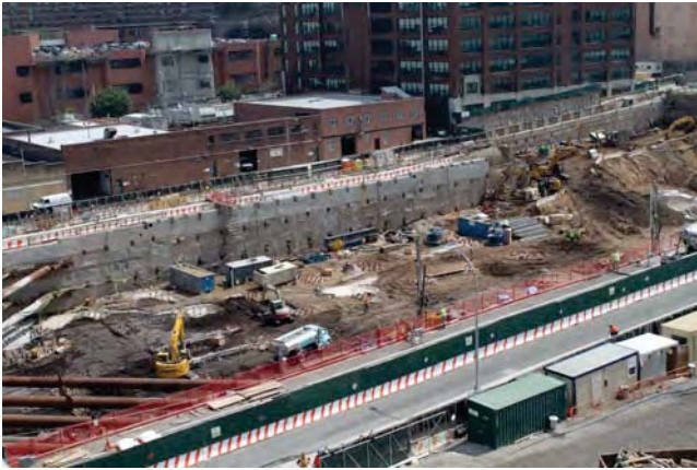
Phase 2 foundations site, looking northeast
