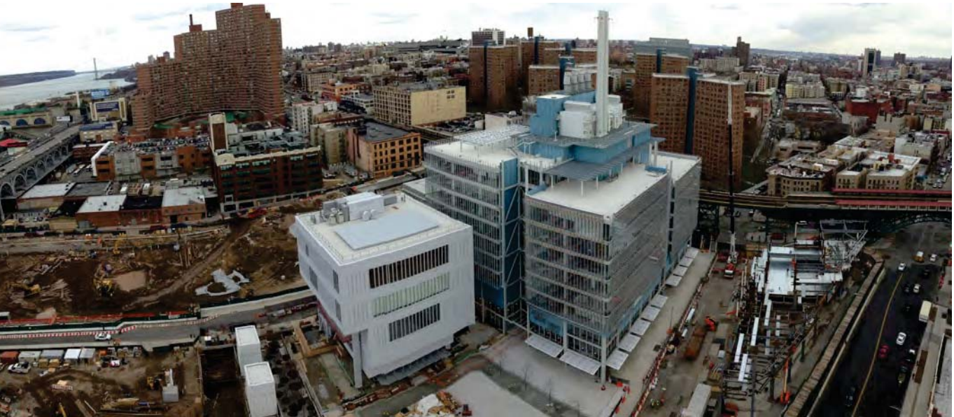
Aerial view looking northeast
