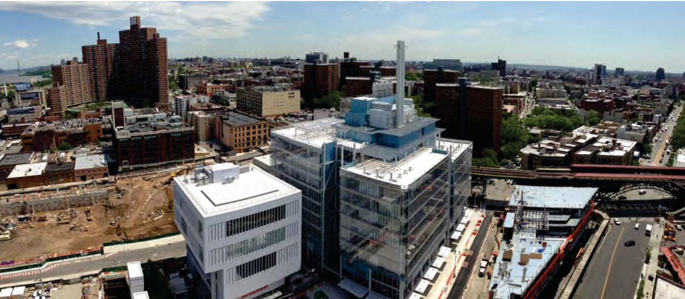
Aerial view looking northeast
