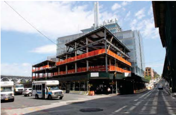
The Forum site, looking northwest
