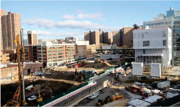
Phase 2 foundations site, looking east
