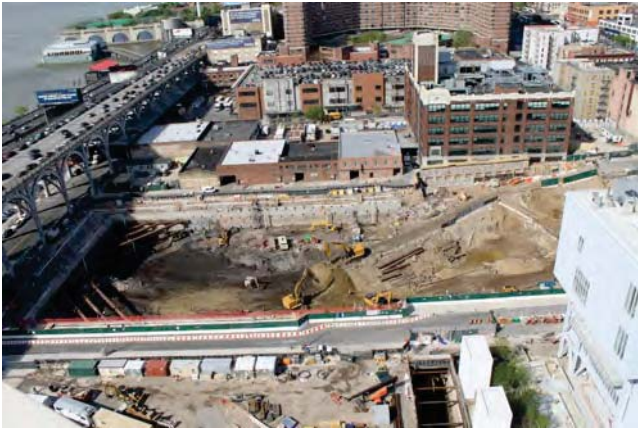
Phase 2 foundations site, looking north
