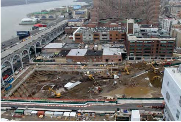
Phase 2 foundations site, looking north
