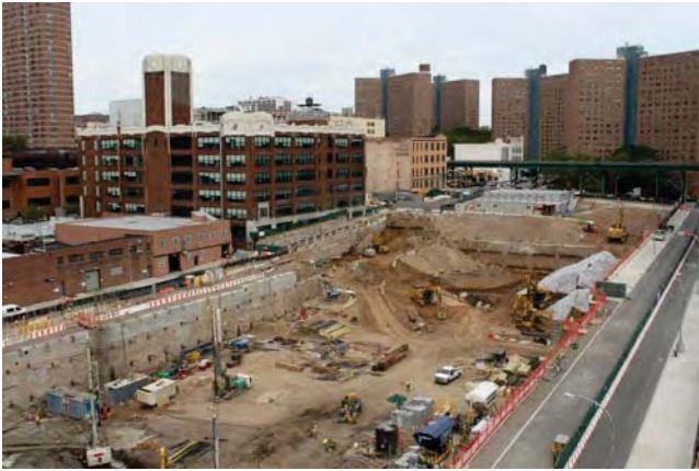
Phase 2 foundations site, looking east
