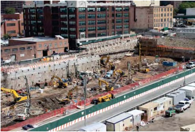
Phase 2 foundations site, looking northeast
