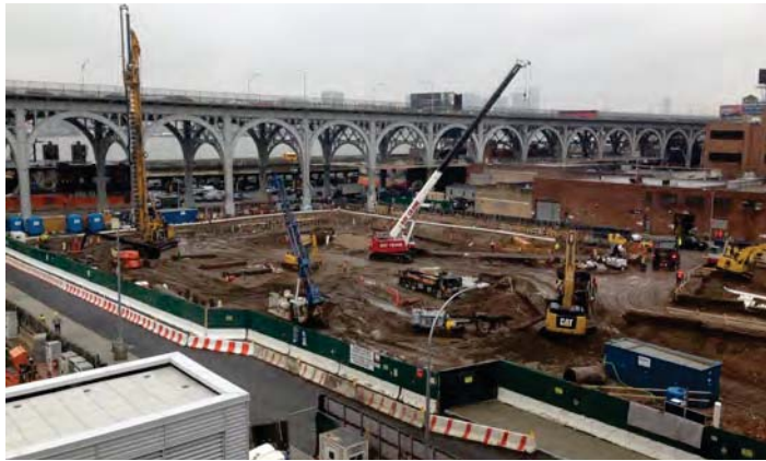
Phase 2 foundations site, looking west
