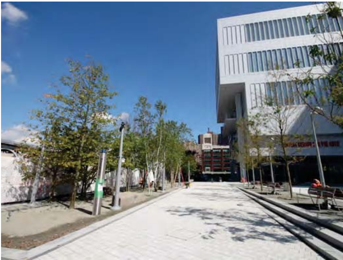
Woodland Walk north-south passageway to the west of the Lenfest Center for the Arts
