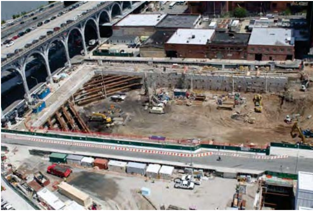
Phase 2 foundations site, looking north
