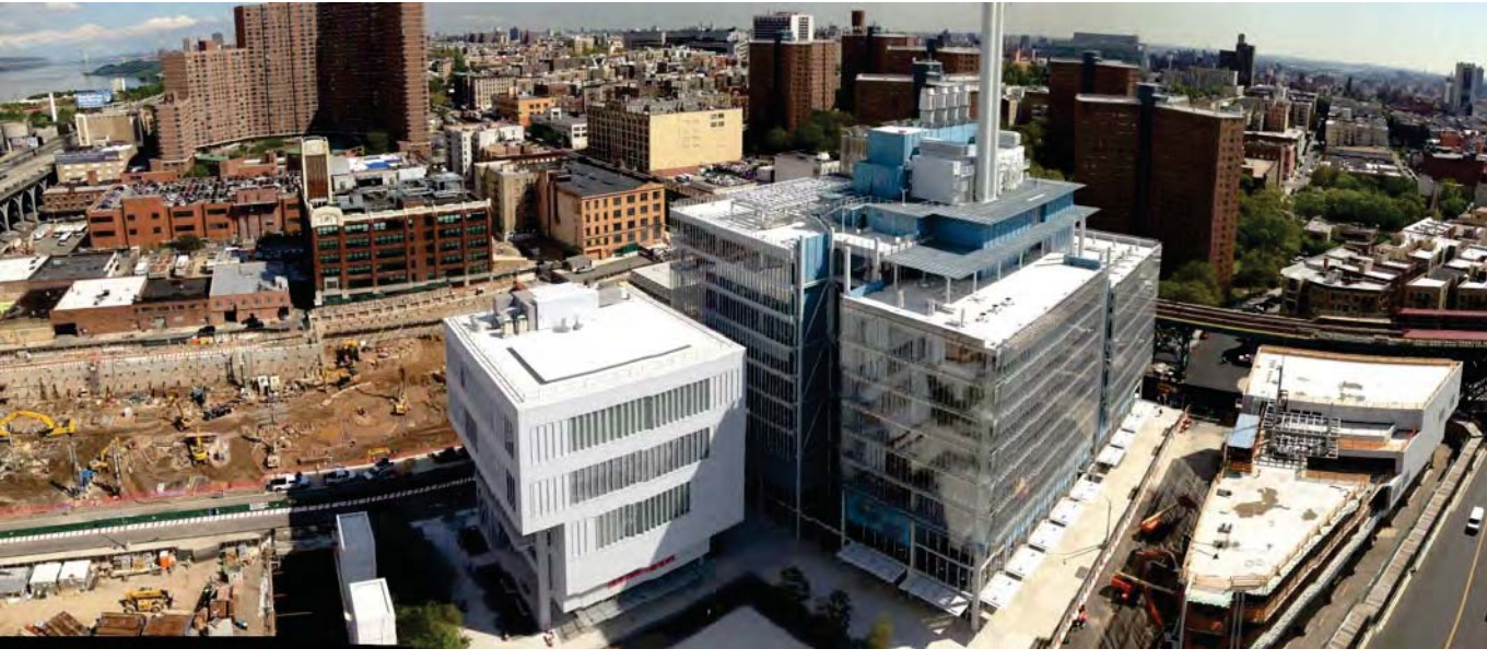
Aerial view looking northeast
