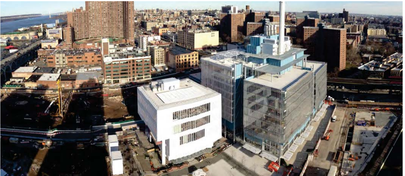
Aerial view looking northeast
