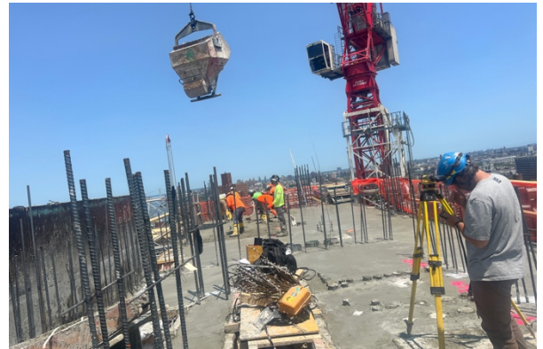
The 34th Floor of 600 W. 125th Street
