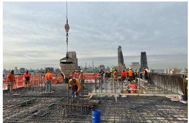
The 22nd floor at 600 W. 125th Street
