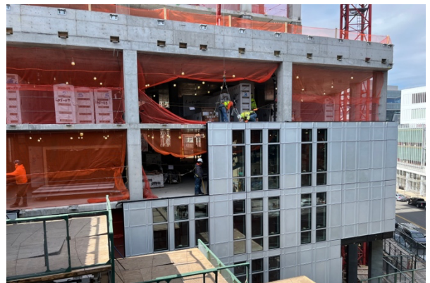
600 W. 125th Street, looking west
