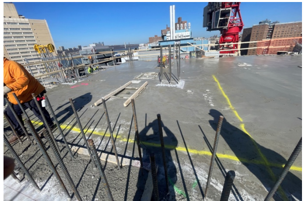
The 15th floor of 600 W. 125th Street
