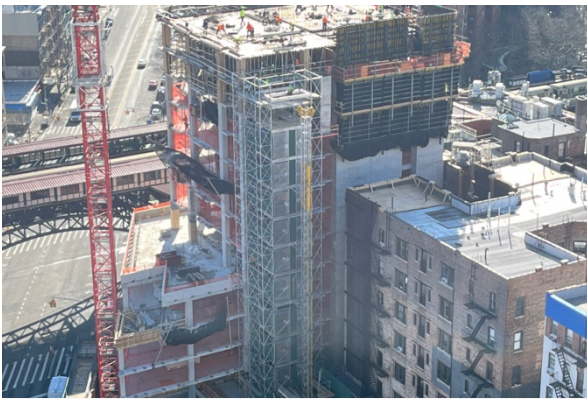
600 W. 125th Street, looking east
