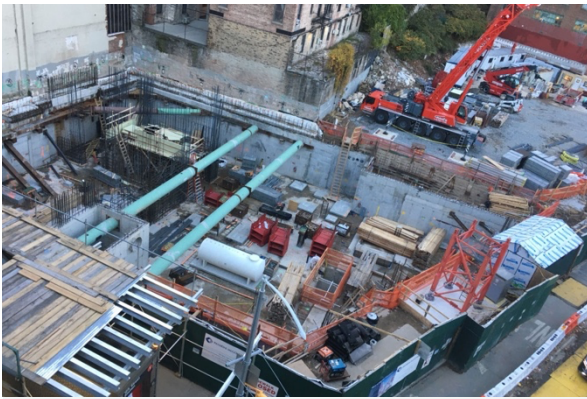
600 W. 125th Street, looking west
