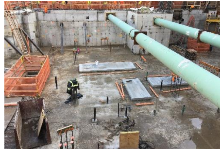
Cellar level at 600 W. 125th Street
