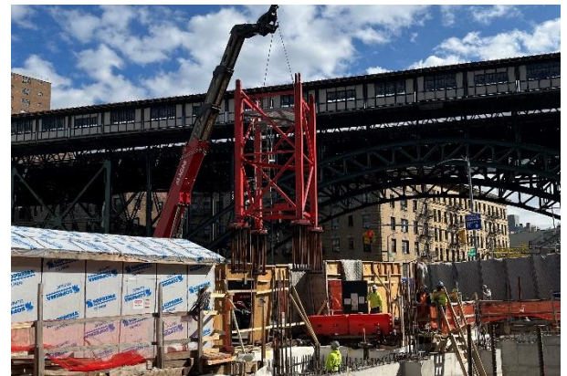
Installation of tower crane at 600 W. 125th Street
