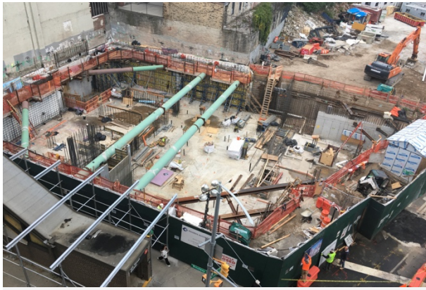
600 W. 125th Street, looking west
