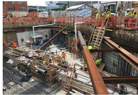
Northern foundation wall at 600 W. 125th Street
