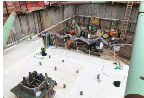
Waterproofing at 600 W. 125th Street
