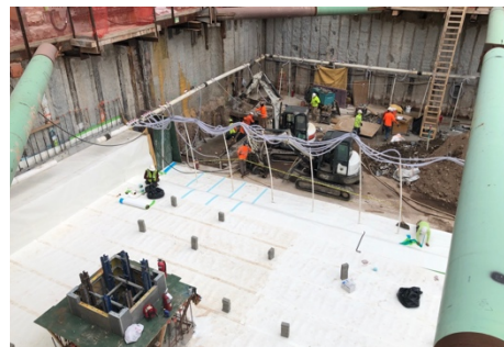
Waterproofing at 600 W. 125th Street
