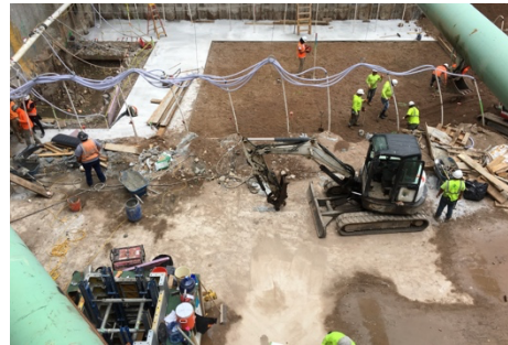
Elevator pit and dewatering system at 600 W. 125th Street
