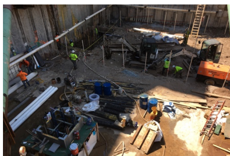
Ejector pit and dewatering system at 600 W. 125th Street
