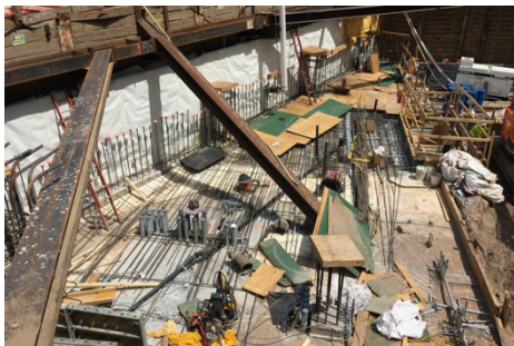
Northern foundation and utilities work at 600 W. 125th Street
