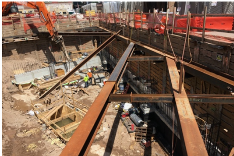
Bracing and foundation work at 600 W. 125th Street
