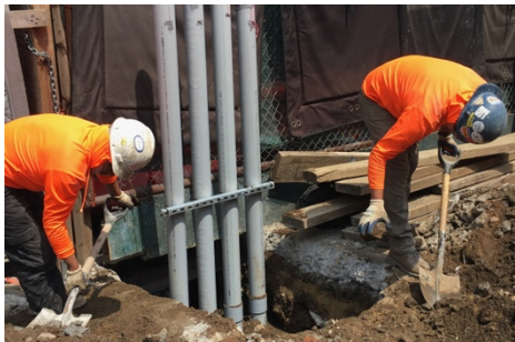
Temporary power conduits at 600 W. 125th Street
