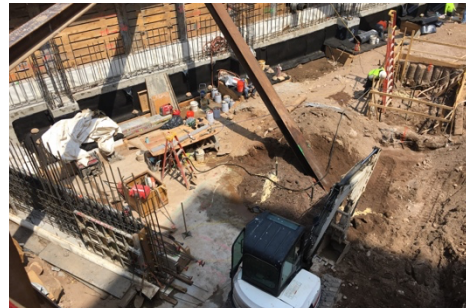
Foundation work at 600 W. 125th Street
