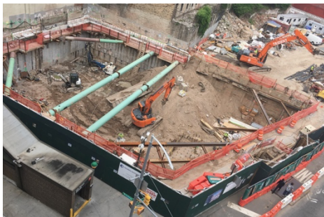
600 W. 125th Street, looking west
