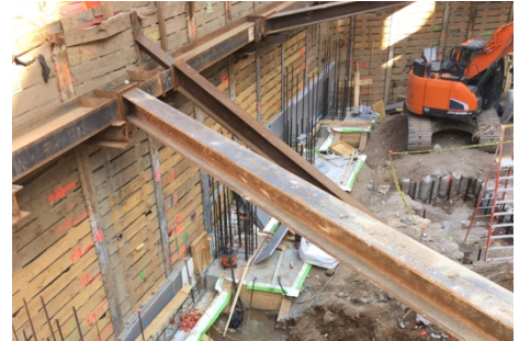
Footing Rebar Installation at 600 W. 125th Street
