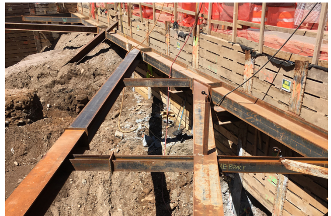
Tangent pile drilling
