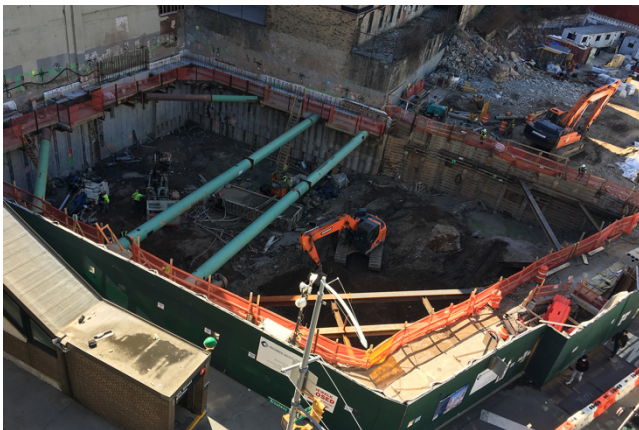
600 W. 125th Street, looking west
