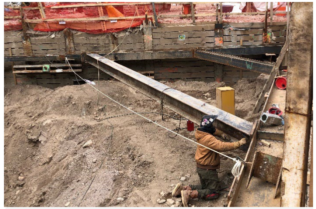
Corner bracing performed at 600 W. 125th Street
