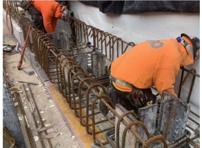
Capbeam installation at 600 W. 125th Street
