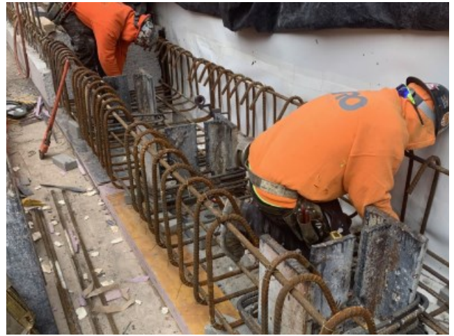
Capbeam installation at 600 W. 125th Street
